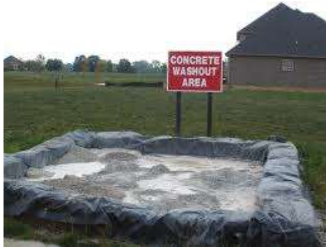
Figure 5.6 Example of temporary concrete washout area
