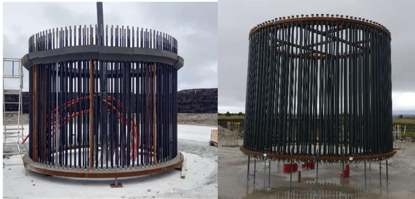
Figure 3.3 Levelled turbine tower can (left) and steel reinforcement being added (right)
