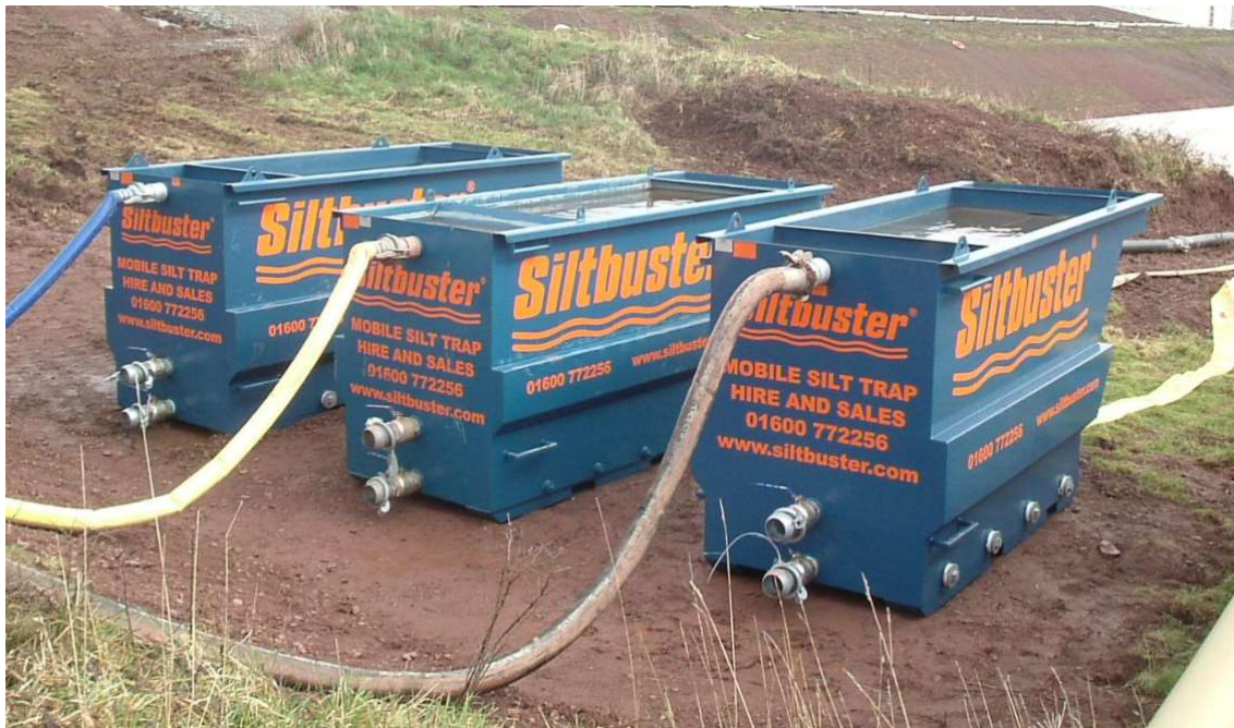
Figure 5.3 Temporary site settlement tanks (Source: Siltbuster)
